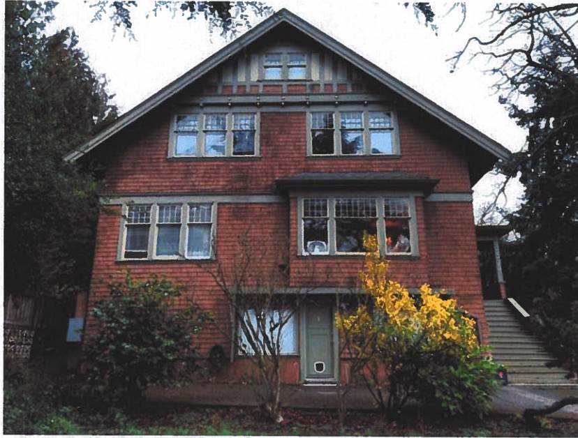
3579 Quadra Street – front: from the west
