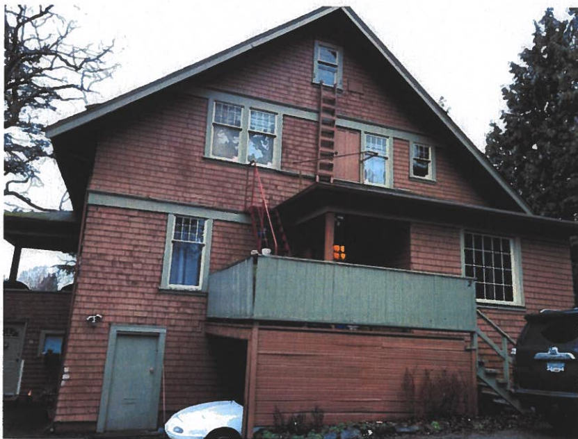
3579 Quadra Street: rear elevation
