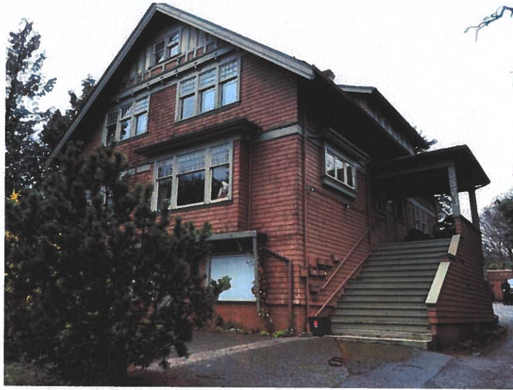
3579 Quadra Street – from the southwest, showing half-timbering and brackets
